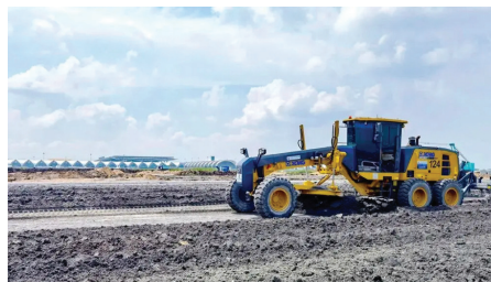
Site Preparation for Buildings
